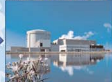
Point Lepreau 680 MWe In-service: 1983
