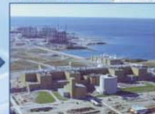
Bruce A 4 unités 900 MWe In-service: 1977-79
