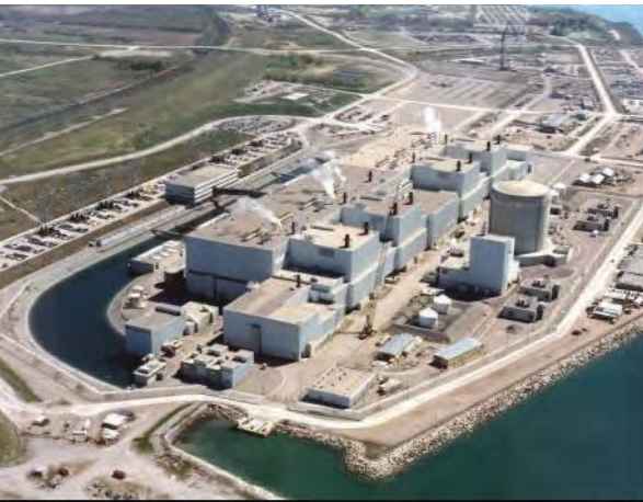
Ontario Power Generation's Darlington nuclear station in Clarington, Ontario.
